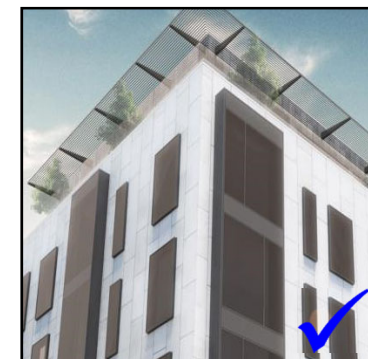
Figure 3.58 Rowdah Apartments, Arabia – Fixed exterior tinted glass overhangs help to reduce solar heat gain while allowing daylight into the interior spaces.
