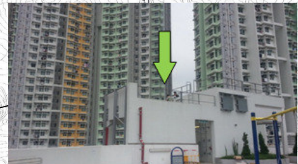
Air Quality Monitoring Station AA1 (Rooftop of Ching Long Shopping Centre)
