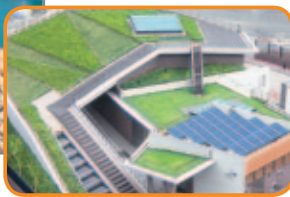
位於太子道東的污水泵站 Sewage pumping station at Prince Edward Road East
