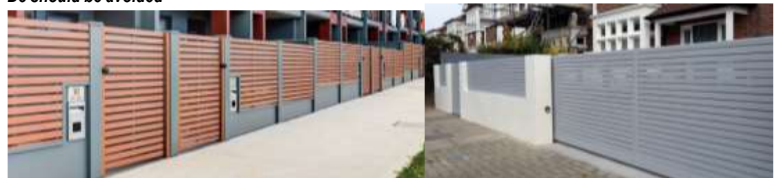
Figure 3.84 Example of zero permeable boundary wall
