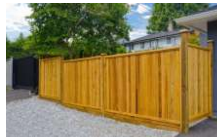
Figure 4.22 Lack of porosity and inappropriate material use
