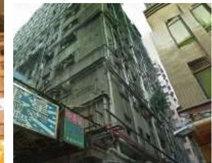
Figure 4.12 piping should not be clear to view
