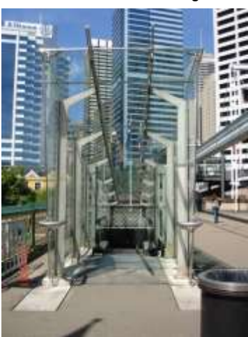
Figure 3.36 Escalator with clear canopy
