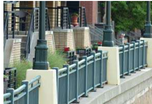
Figure 4.13 Visually porous fence walls enhance openness and visual permeability.
