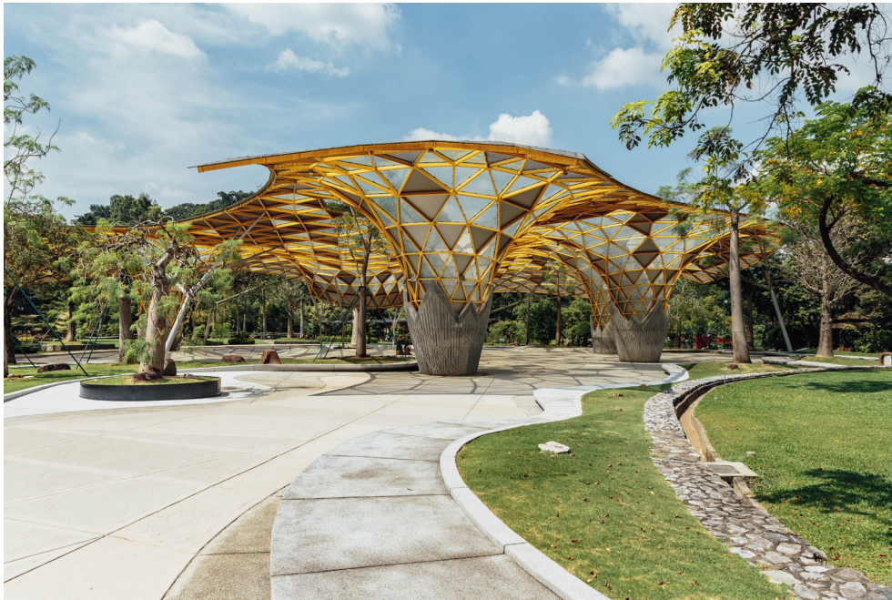
Fig. 3-28 History - Aviation theme employed in the choice of building materials and character of design elements Perdana Botanical Gardens, Kuala Lumpur [Source: Shutterstock]
