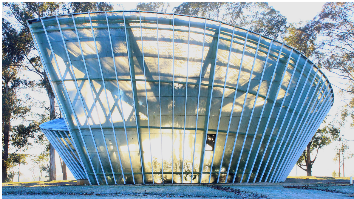
Fig. 3-29 Use of metal, glass, concrete and timber as combination of materials for building structures Top: ArchSD Public Toilet, Tin Shui Wai Park Bottom: [Source: Shutterstock]
