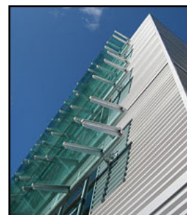
Figure 3.80 The Terry Thomas building, Seattle – Fixed exterior tinted glass overhangs help to reduce solar heat gain while allowing daylight into the interior spaces.
