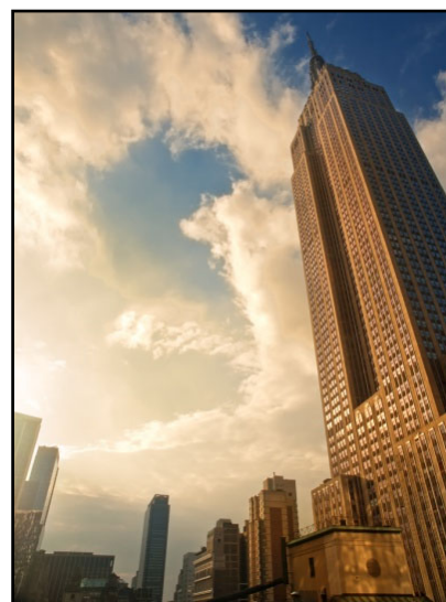
Figure 3.76 The Empire State Building, New York: An office building with a history that anchors itself as an icon of leadership for the world. The ground breaking energy efficient retrofitting has cut $7.5M in energy costs over the past three years.
