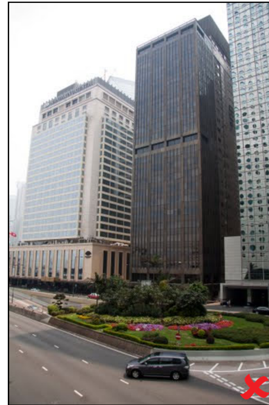
Figure 3.86 Dark glazed buildings can produce a gloomy internal and external atmosphere
