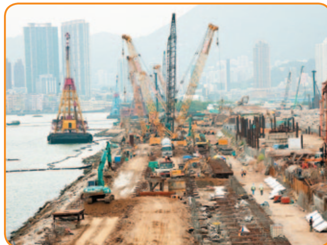
郵輪碼頭土地平整工程 Site formation works for cruise terminal
