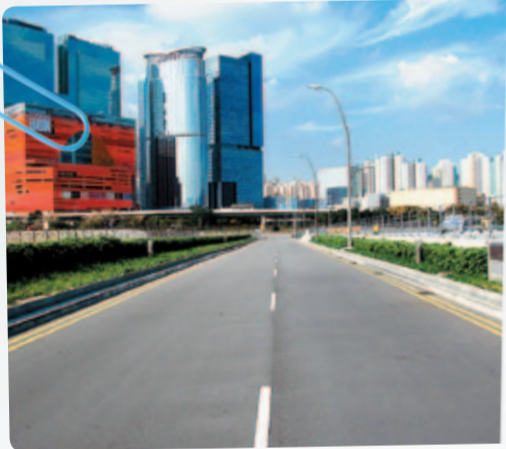
改善後的前飛機滑行道橋樑 Enhanced Former Taxiway Bridge
